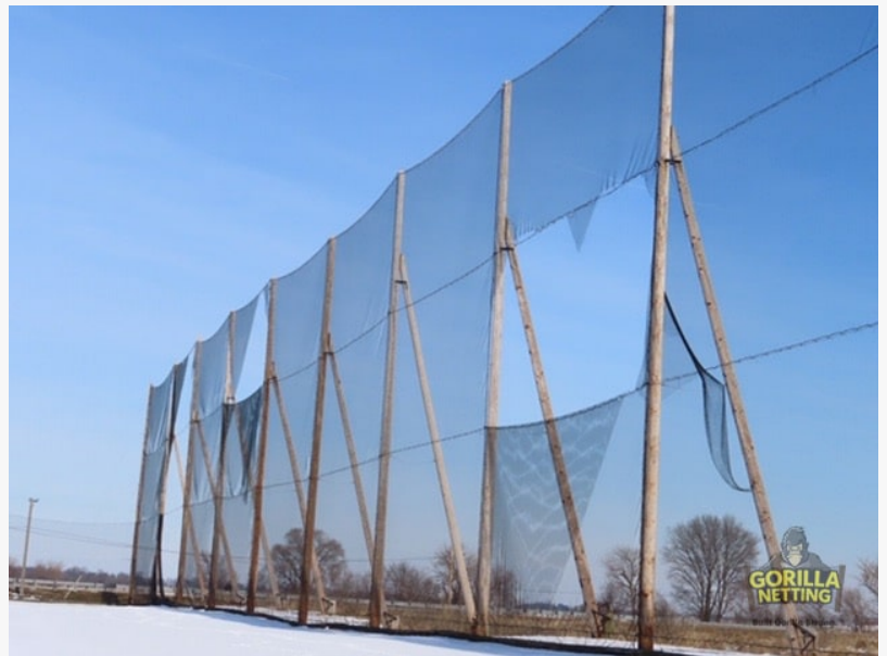
The damaged driving range netting system at Sugar Grove Golf Center before replacement
