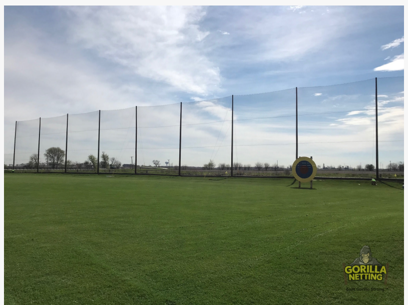
The newly replaced driving range netting system featuring a much cleaner look with the new netting and down guy replacements.
