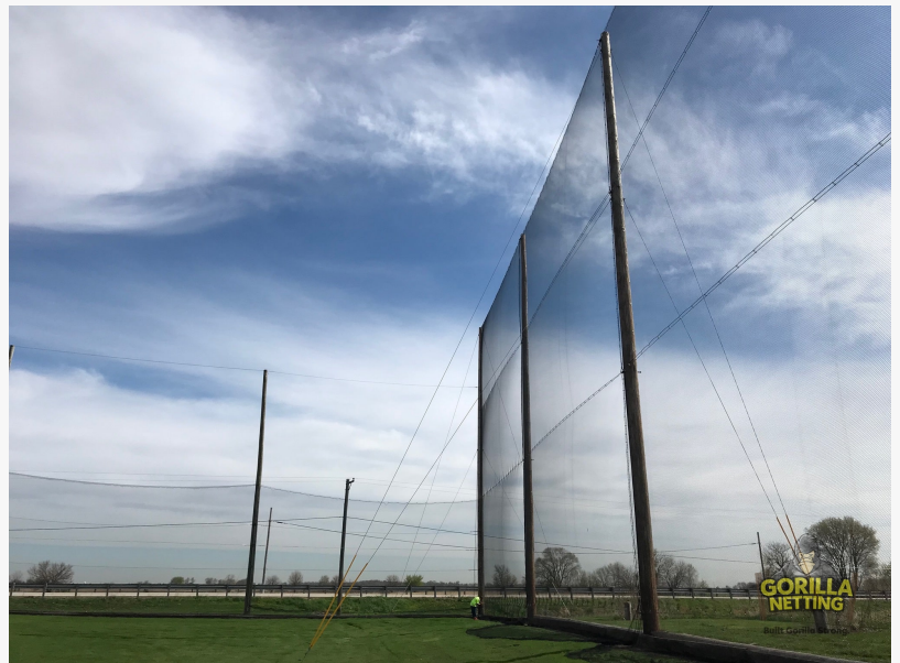
New netting panels and down guys replace damaged netting and push poles.
