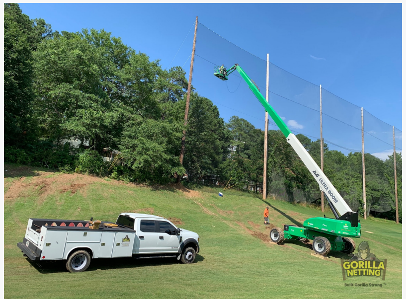
Netting Contractor installing the extension of the netting panels at The First Tee of Atlanta.
