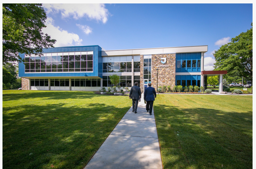
Jefferson Institute for Bioprocessing facilities
