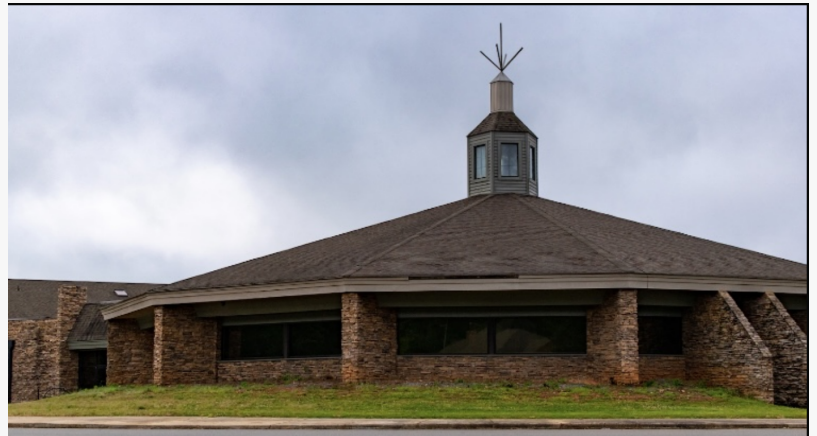
The Longhouse, the Catawba Government headquarters where the vote took place last February 19th.
