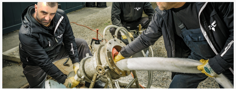
Sewer cleaning Antoniou
