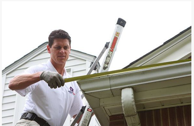
HandyPro fixing gutters
