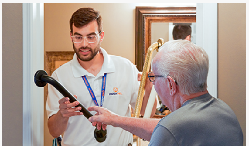
HandyPro installation bathroom safety
