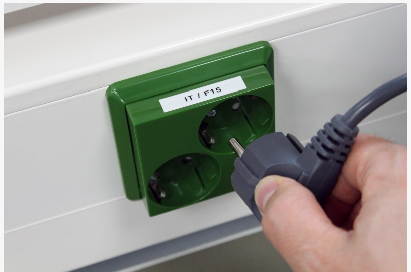
The staff have localized and replaced the faulty device.
