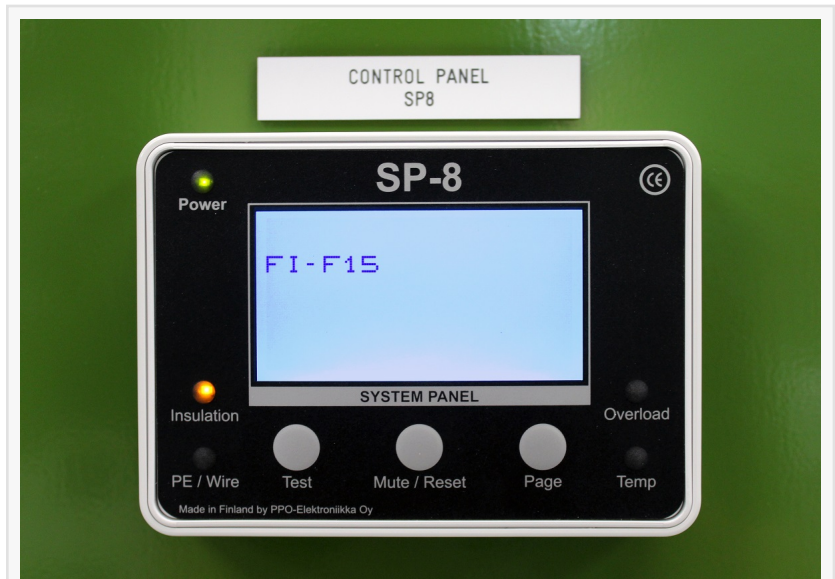
Insulation fault in the socket F15
