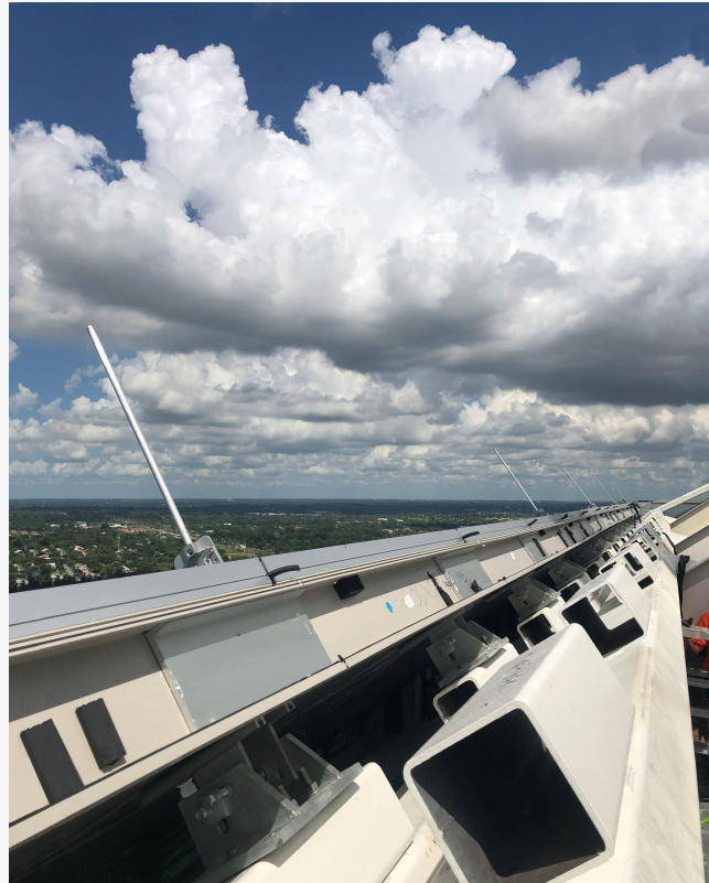
Lightning protection system installed on the Hard Rock Hollywood Resort and Casino
