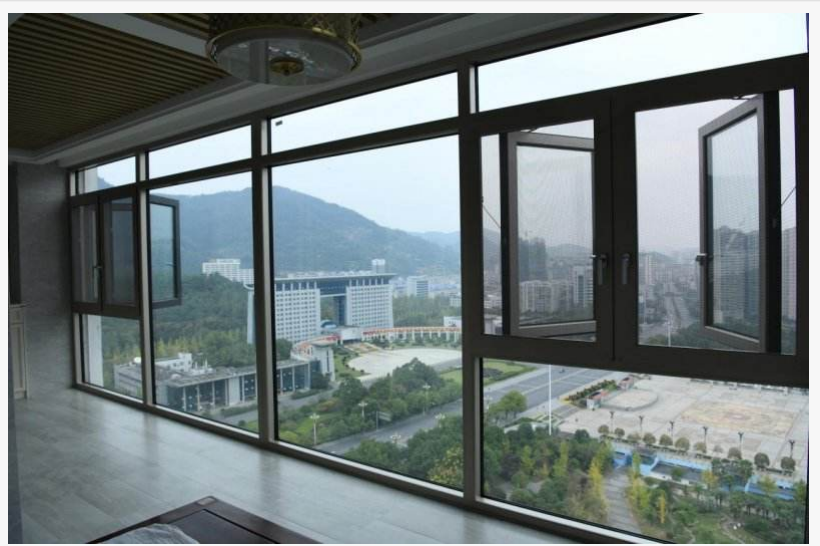
Thermal-break-aluminium-windows-is-becoming-thick-and-heavy-to-get-better-energy-efficiency
