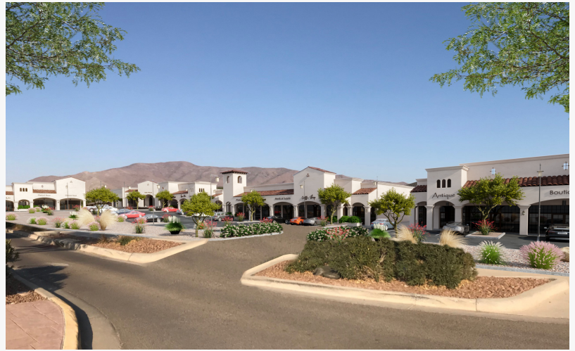
Paseo Del Norte Medical / Office/ Retail Project
