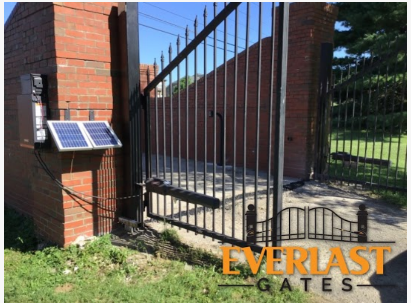
Solar Operated Gate Installation
