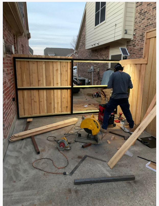
New Gate Install
