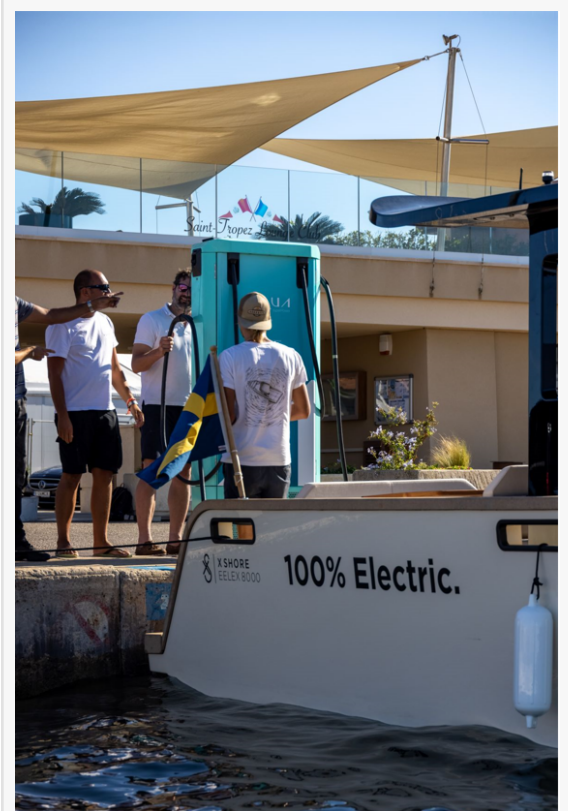
The Aqua 75 rapid charging the X Shore Eelex 8000 (Credit Aqua superPower Ltd)
