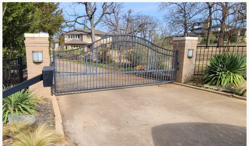
Southlake - New Gate Install
