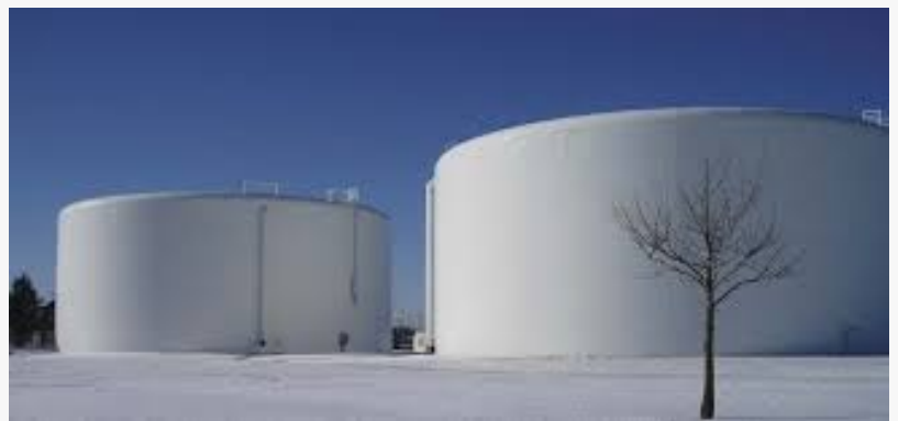
Potable Water Tank Coatings
