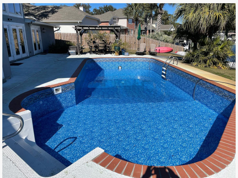
Pensacola Swimming pool liner replacement
