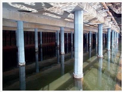
One of the most extreme environments for steel corrosion is sea water. ZINGA protects over 200 immersed steel piles at Killybegs harbour in Ireland
