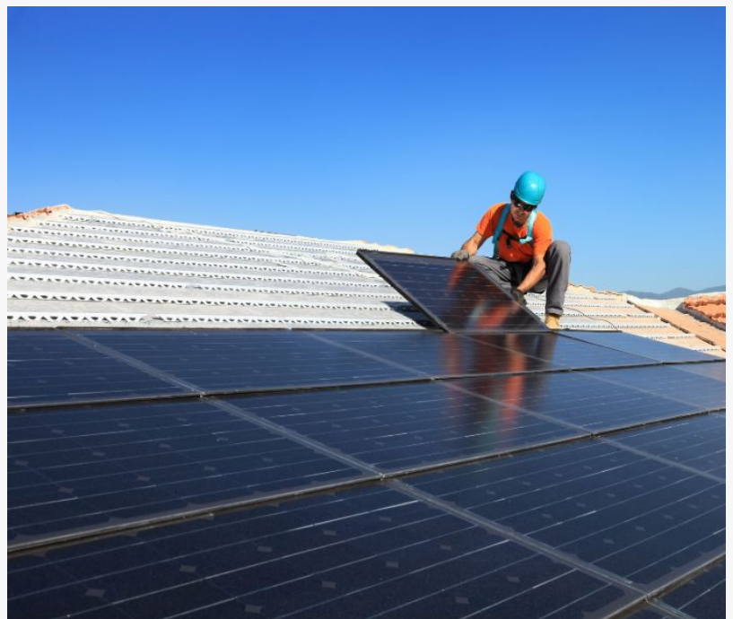
Solar Panel Installation for Texas Home
