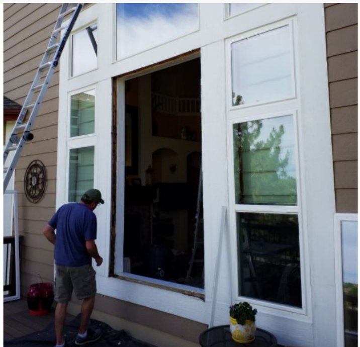
Crew installing a window in McKinney
