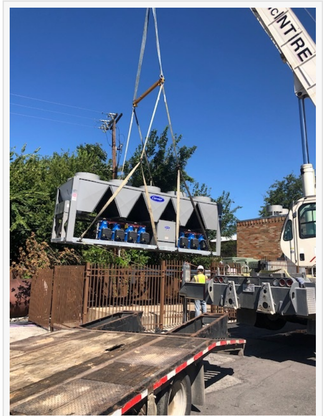
Estrella iPlant Installation
