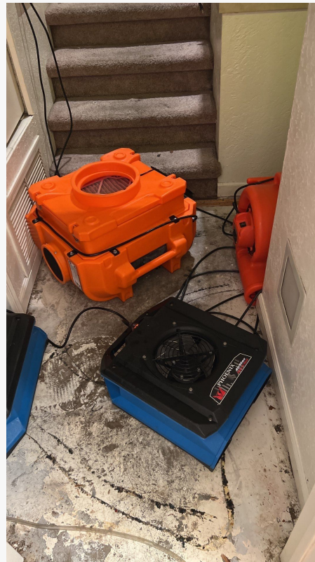
Dry out equipment set up to dry out walls and flooring after water damage from a toilet.
