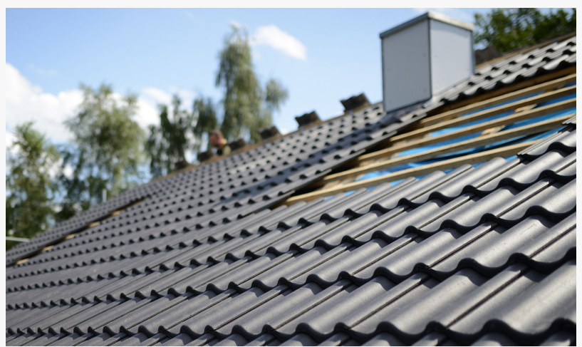
Montclair roofers - roofing
