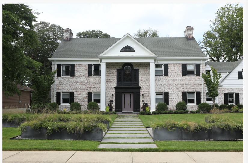
Montclair Roofing - roofing services
