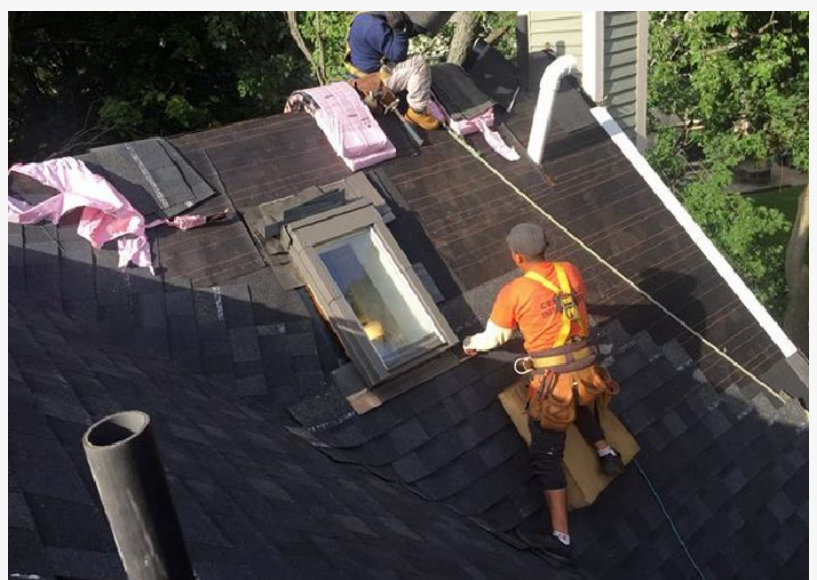
roof repair job in Warwick
