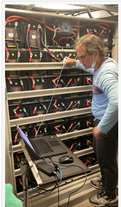
Umer Anwer, Urban Electric Power's VP for Systems Engineering, during installation
