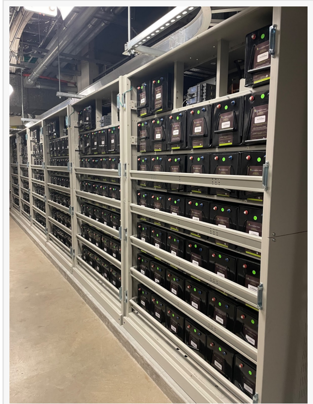
A portion of the San Diego Supercomputing Center’s new power backup system
