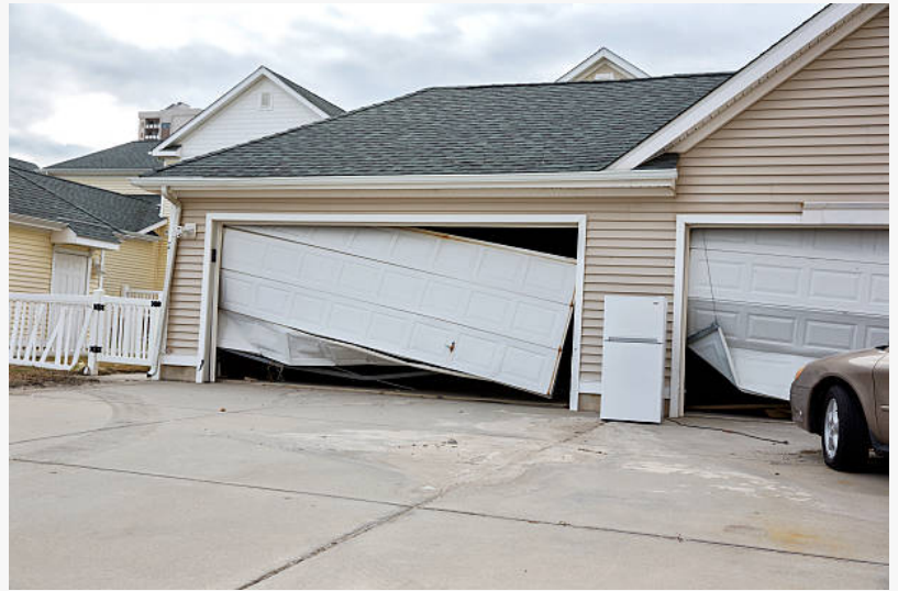
Emergency Garage Door Services Mankato MN
