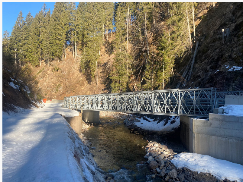
Acrow Bridge - Alps Italy
