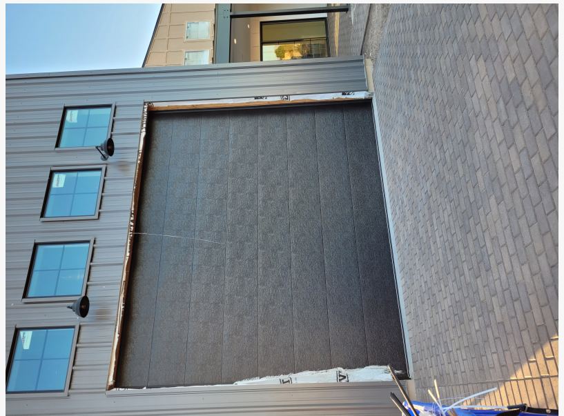
Emergency Garage Door Repair in Mankato MN
