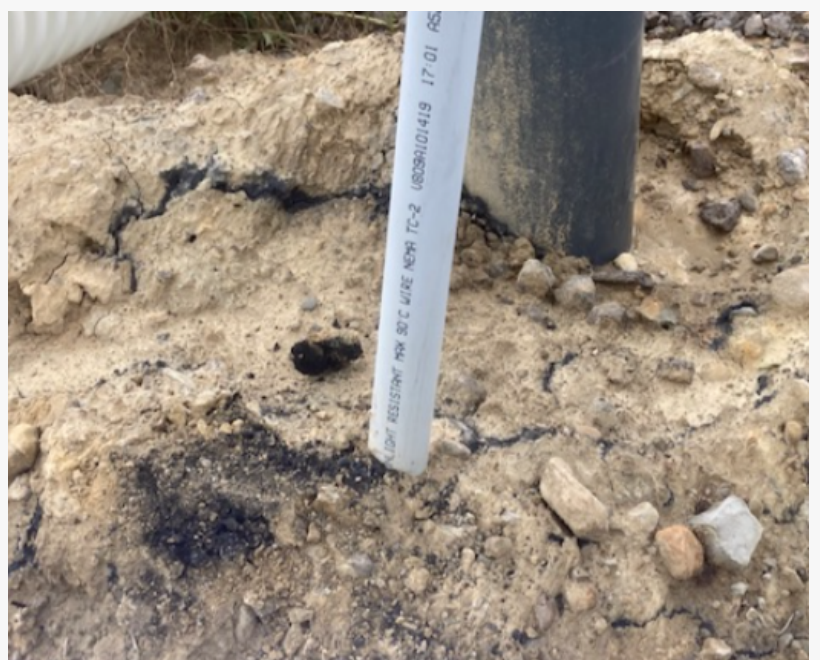
Black "veins" where ultra-concentrated hydrogen sulfide "ate" through the soil barrier at the Lordstown Landfill. Toxic gas pours out of these veins making matters worse.
