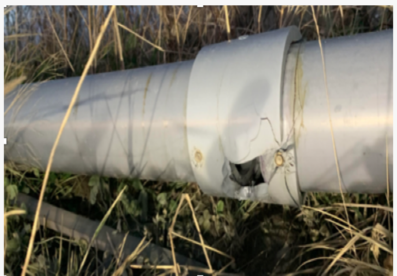
Lordstown Landfill's low-budget gas system has chronic failures. Pipes burst, valves and control systems malfunction allowing highly concentrated toxic gases to escape.
