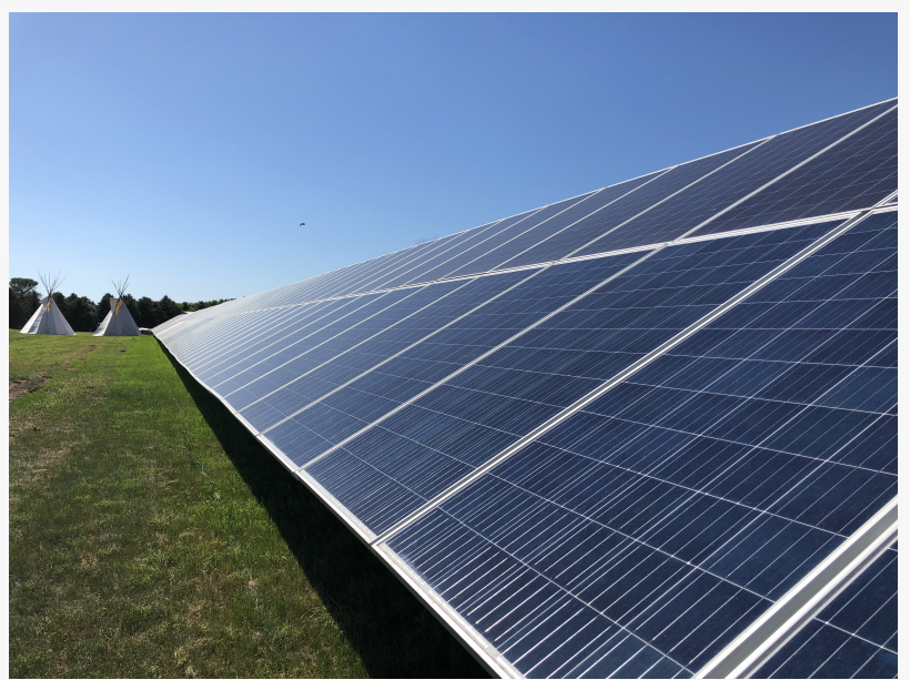
300kW community solar farm for Standing Rock Sioux
