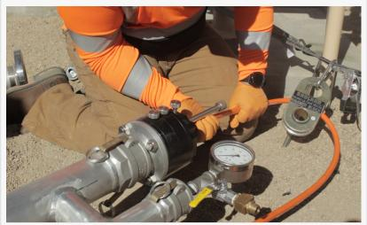
The County's force main will be surveyed without disruption of service and without temporary bypass pumping using Electro Scan's pressurized insertion tube.
