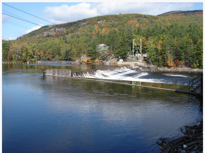
Gorham Dam, located in Gorham, NH, is one of CRP's first two above 1MW hydro facilities approved by the NH DOER to participate in Group Net Metering set to begin benefit flow today.
