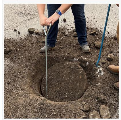
Electro Scan's readings automatically detect buried manholes, as found in Austin, Texas, not included on GIS.
