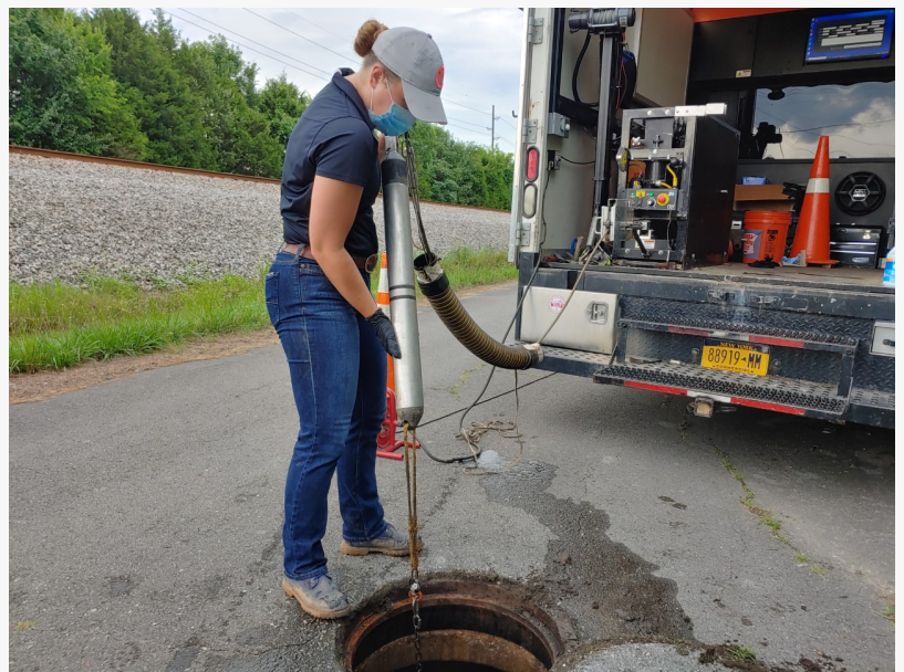
Mackenzie App, VP Product Management, Gravity Pipelines,, Electro Scan Inc. inserts ES-620 probe into sewer main.
