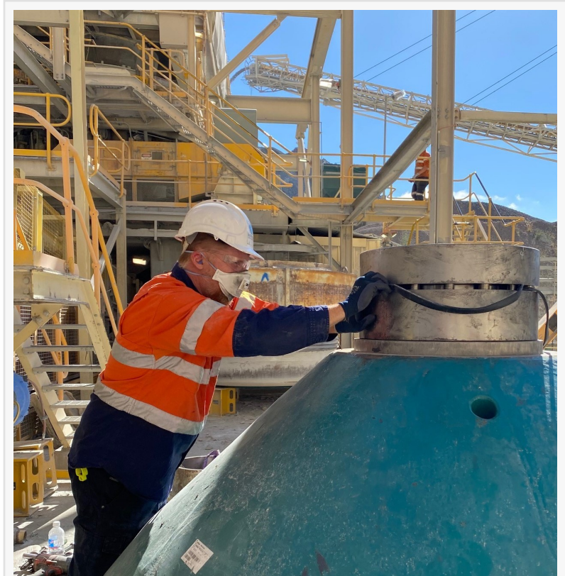
Technofast’s EziTite Hydraulic Head Nut being installed on a gyratory crusher
