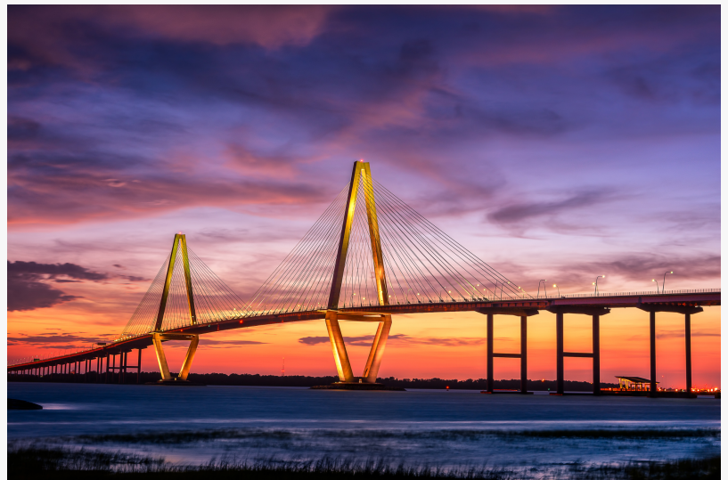
Charleston, South Carolina
