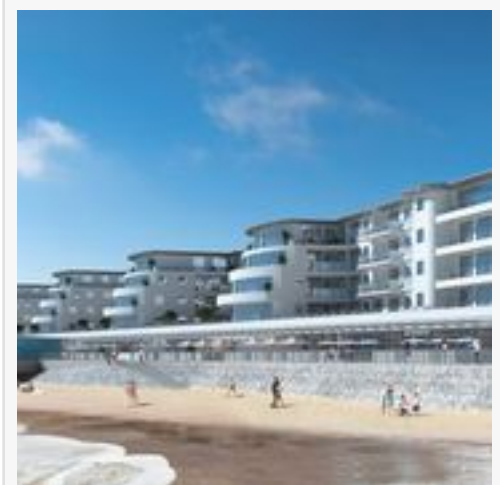
Royal Sands Ramsgate development adjacent to Ramsgate Royal Harbour yards from the beachfront
