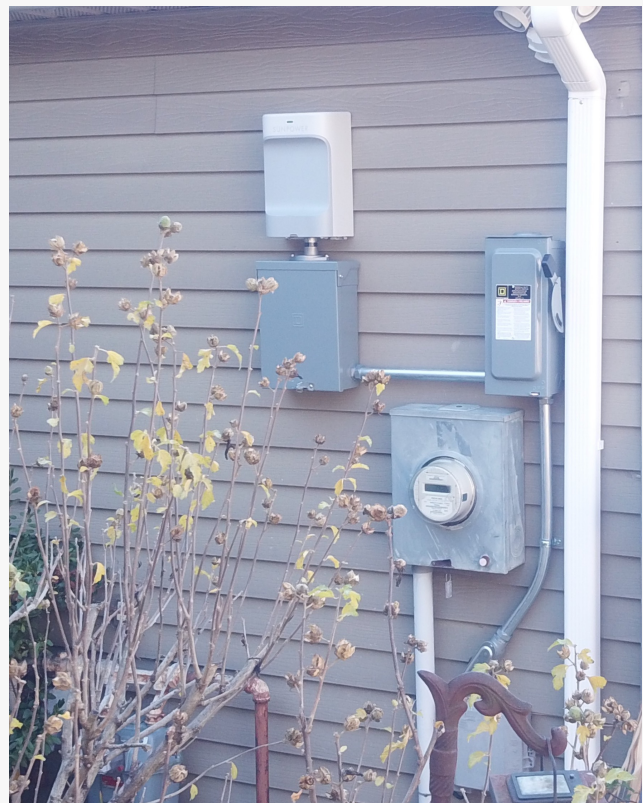
Award Winning Inverter and Meter Installation
