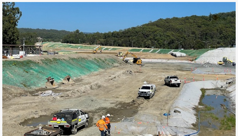
RST Solutions' advanced soil binder Total Ground Control applied to batters and embankments to reduce dust and erosion
