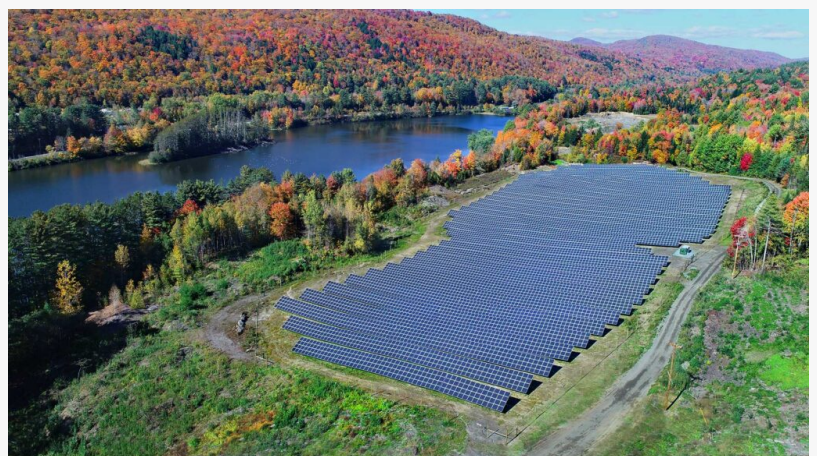
New solar array in Hardwick, VT
