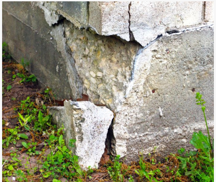
foundation repair for a Bloomington IN home
