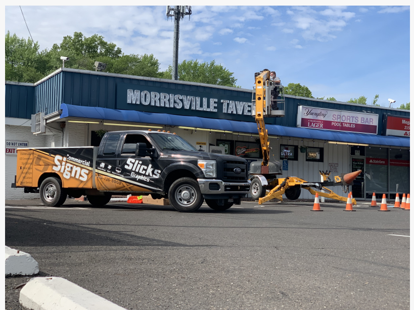
Completing the Morrisville Tavern sign installation.
