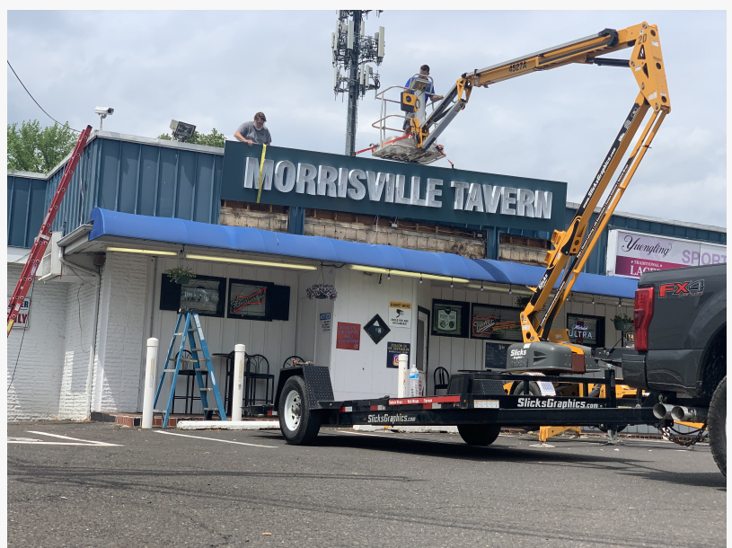
Slicks Graphics installing the new Morrisville Tavern Sign
