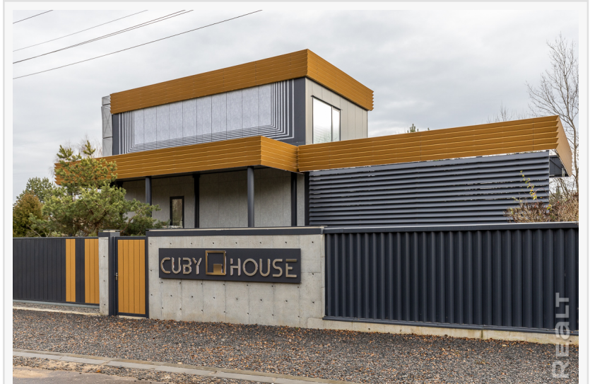
First house built with Cuby Technologies
