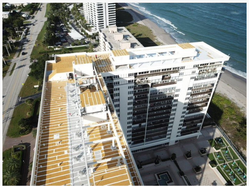
Commercial Roofing Project E.W. MacDowell Inc. Wellington, Florida
