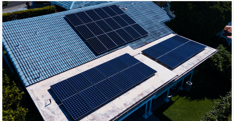
Residential Solar Installation on Oahu
