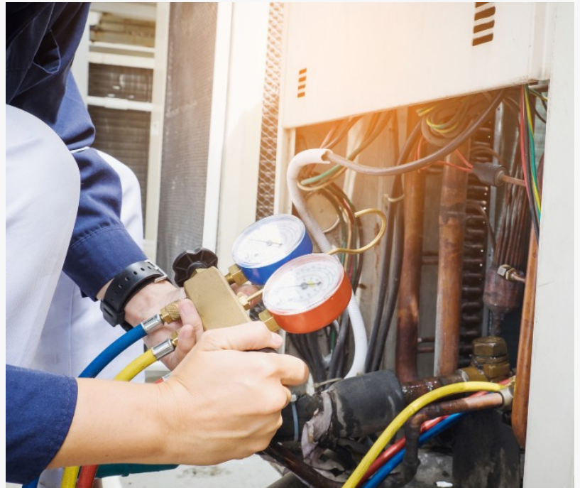
AC repair for a home in Humble, TX
