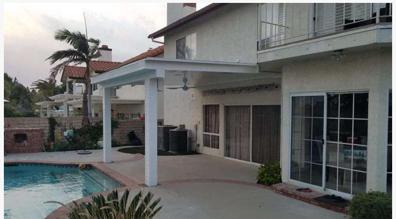
Vinyl Patio Cover in Los Angeles
