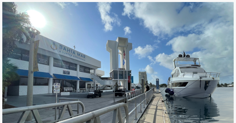
Aicon yacht dockside with Hydrogen station for on-board Renewable Innovation's Hydrogen Fuel Cell systems at Bahia Mar Marina, Fort Lauderdale, FL
