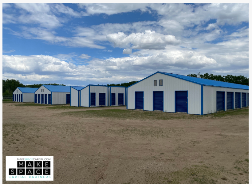
Make Space™ Storage - Prince Albert
