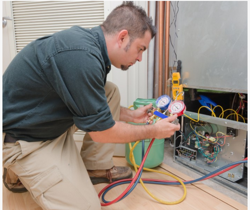
AC repair service in Humble, TX
