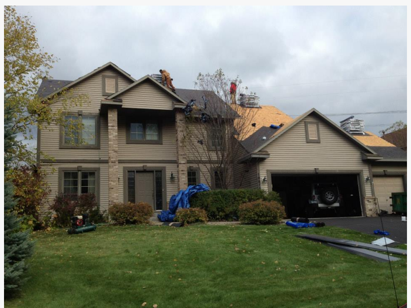
Liberte Construction Roofing Installation Fridley
