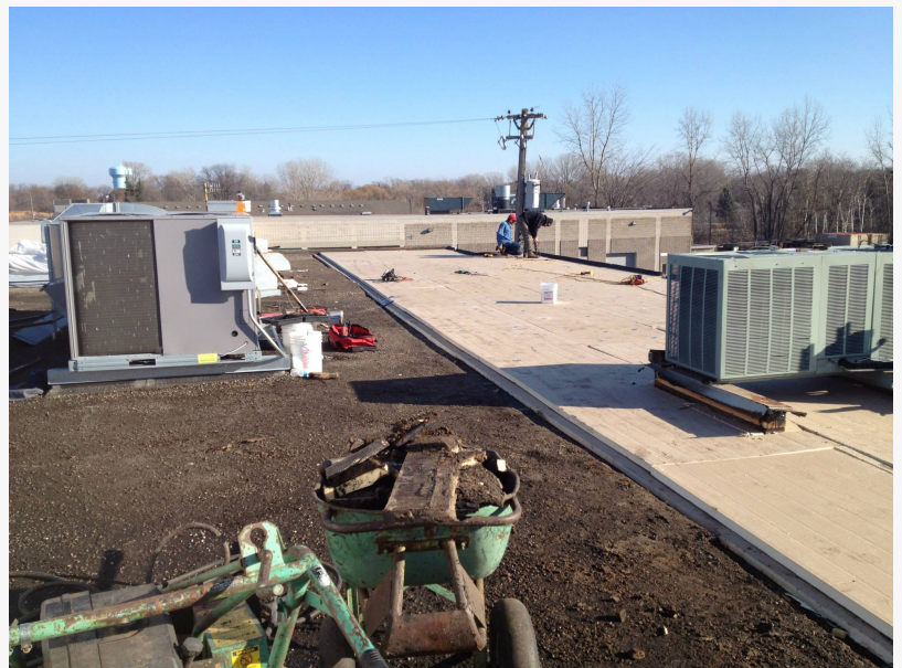
Liberte Construction Commercial Roofing St Cloud
