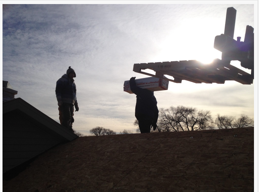
Liberte Construction Roofing Repair New Hope
