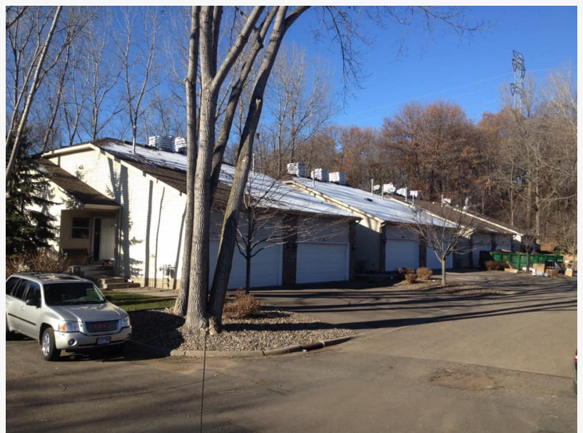
Liberte Construction Roofing Installation Minneapolis
